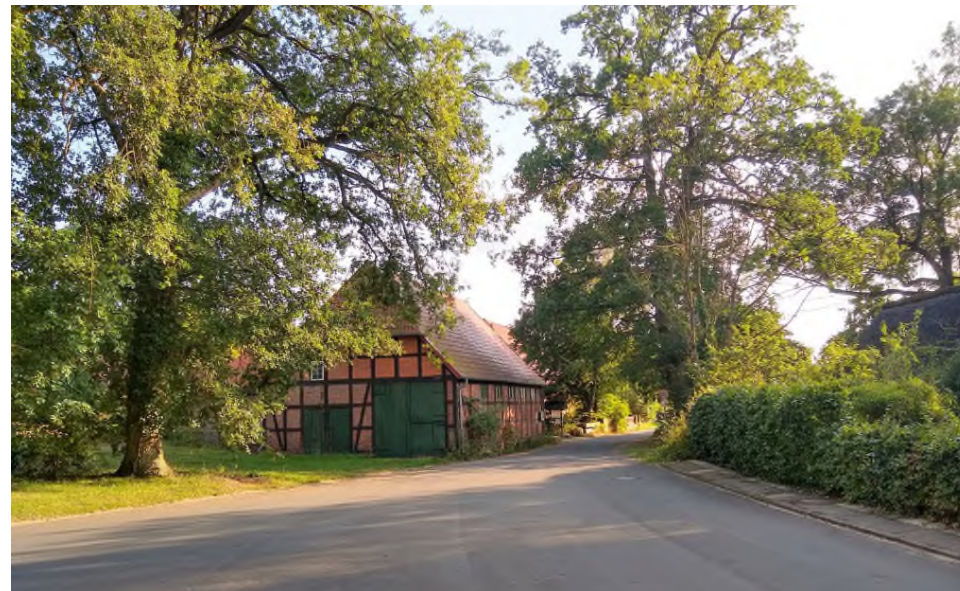
Abb. 17 Scheune in Radenbeck
